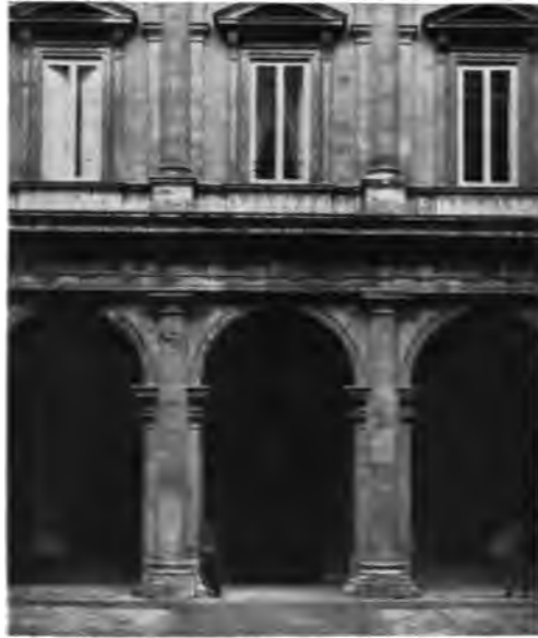
A TYPICAL ARCH-AND-COLUMN COMPOSITION OF THE ITALIAN RENAISSANCE, BASED ON THE ROMAN USE OF ARCH AND COLUMN (Courtyard of the Farnese Palace, in Rome)
